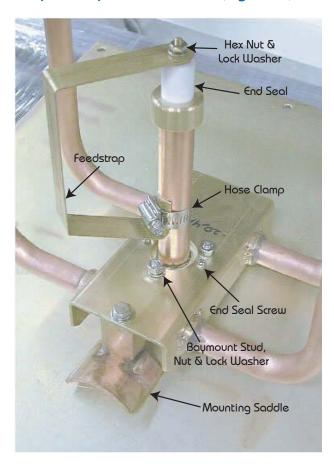
a. On each bay, remove the hex nut, lock washer, and hose clamp securing the feedstrap to the end seal, and remove the feedstrap.
